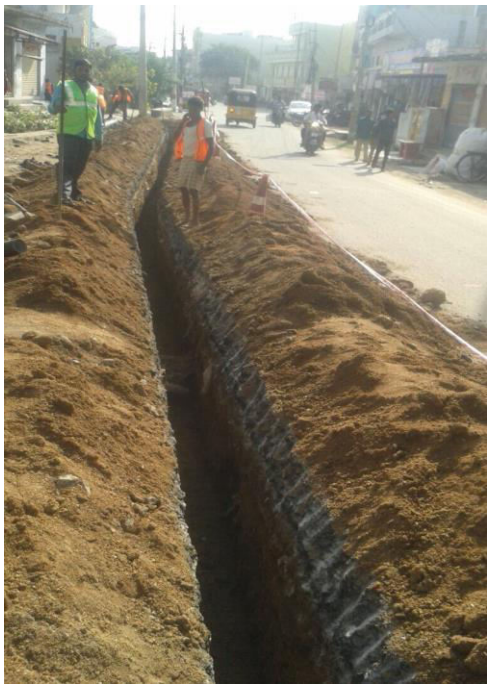
Distribution Network Pipeline Laying
