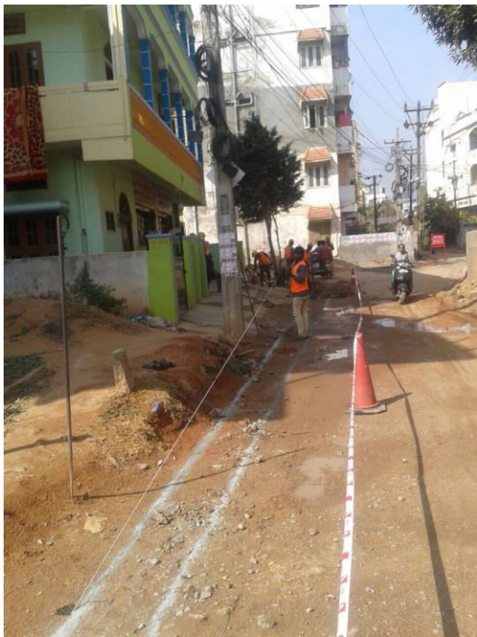
Distribution Network Pipeline Laying
